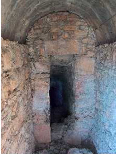
Fig.13: The water duct where it exits the tunnel in the south
